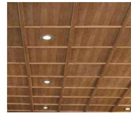
Description: Ceiling Wood Panels Mfr: Custom
